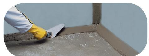
of **weberpremix fiber**. Thickness can reach 15 mm and carry additional 3 days of curing. In case more thickness is required to achieve the alignment, then scratch the finishing coat and apply another one following the previous steps.
