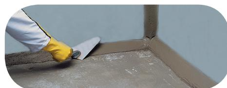
of **weberpremix fiber**. Thickness can reach 15 mm and carry additional 3 days of curing. In case more thickness is required to achieve the alignment, then scratch the finishing coat and apply another one following the previous steps.
