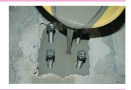
Thoroughly scab the foundation, clean the area between the foundation and machine base-plate, as well as the anchor holes. Build a solid leak-proof formwork. Saturate the concrete foundation with water for at least few hours prior to pouring. Remove all residual water.
