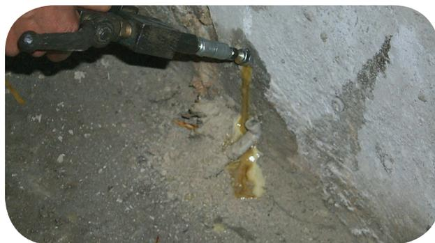
Drill a hole in the concrete at 45 degree angle in order to intersect the crack or the leaking construction joint.
