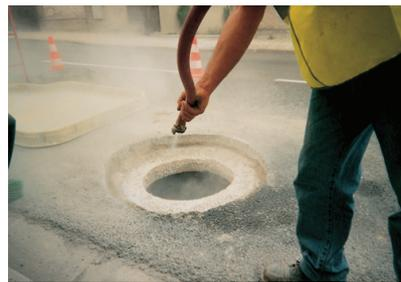
Clean dust and other materials, remove traces of oil, grease, etc... by brush or air-blowing
