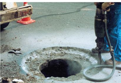
Break and cut 10cm around the manhole at a 90 degrees angle
