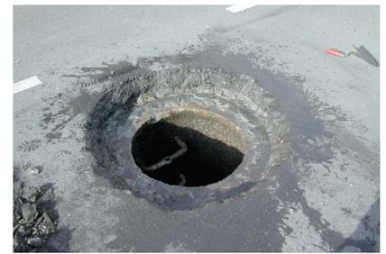
Humidify the area where the mortar will be laid. It should be wet but not waterlogged.
