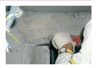
In the freshly casted concrete, superficial damage are revealed as honeycombs with exposed aggregates, pinholes or surface imperfections.
