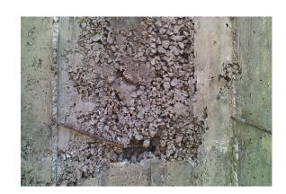
In case of pinholes, surface should be dampened with water to surface saturated dry prior to cementitious repair. In case of using epoxy based products for repair, water should not be used on the surface in any circumstance. The area should be grinded in order to get rid of laitance, paint or any covering material, and then should be cleaned with an air blower.
