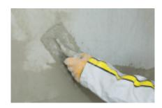
**Conrep.360 FFR** a premixed coating composed of very fine fillers and modified polymers. When mixed with clean water, using an electrical mixer, it turns into a smooth paste. Applied to surface with a trowel, it provides a smooth and velvet-like finish that adjusts superficial irregularities with a thickness up to 3 mm.
