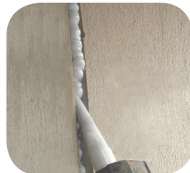
**weber jointseal PU** is a reliable low modulus polyurethane joint sealant, allowing a high degree of elongation after stretching.
