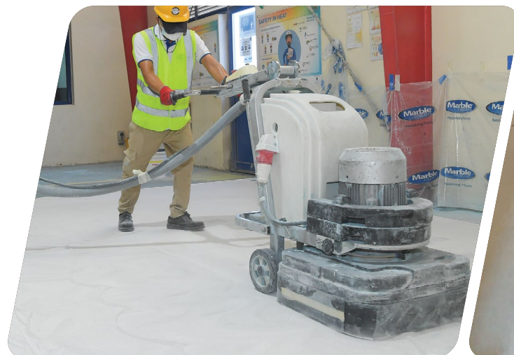
5 Grinding After 24 hours, grind the surface using a heavy duty grinding machine
