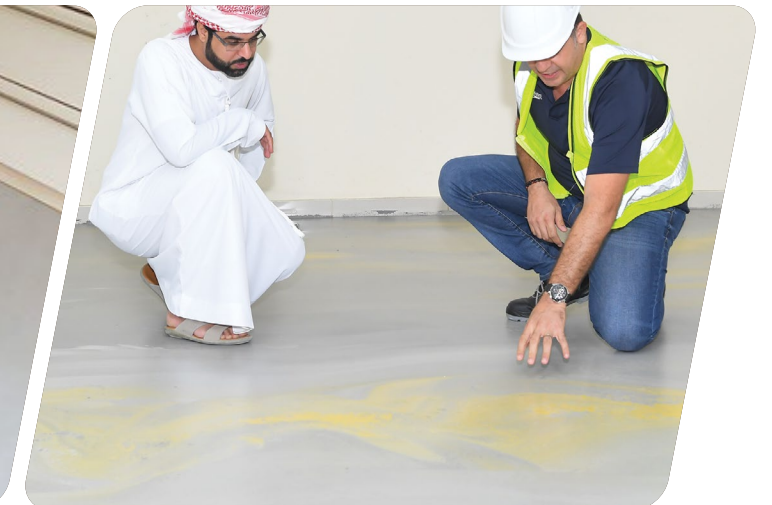
8 Trafficable The floor will be ready to accept light foot traffic after 24 hours
