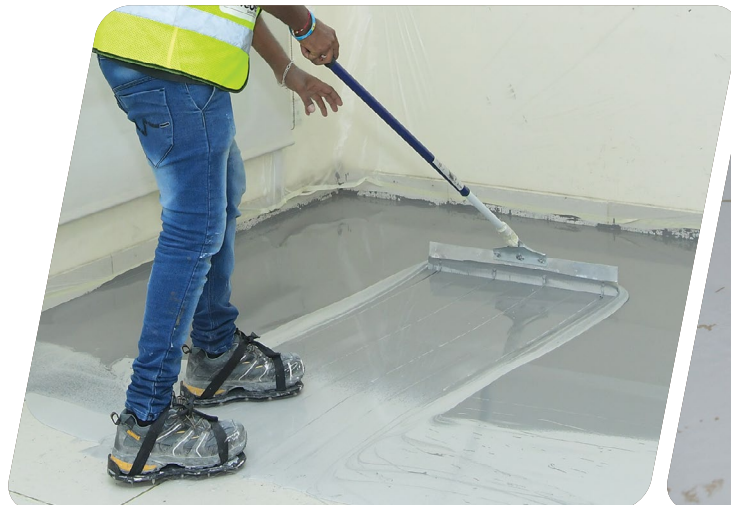
5 Levelling Level the mixture by using a pin leveller
