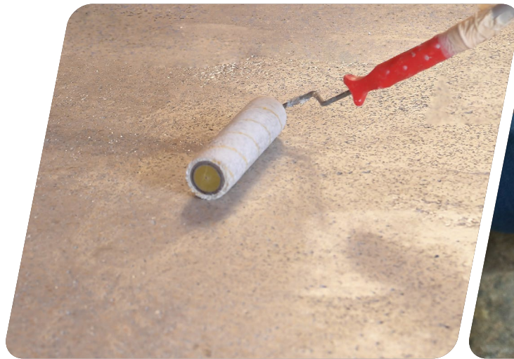
1 Priming Prime the surface using weber euroflor Prime
