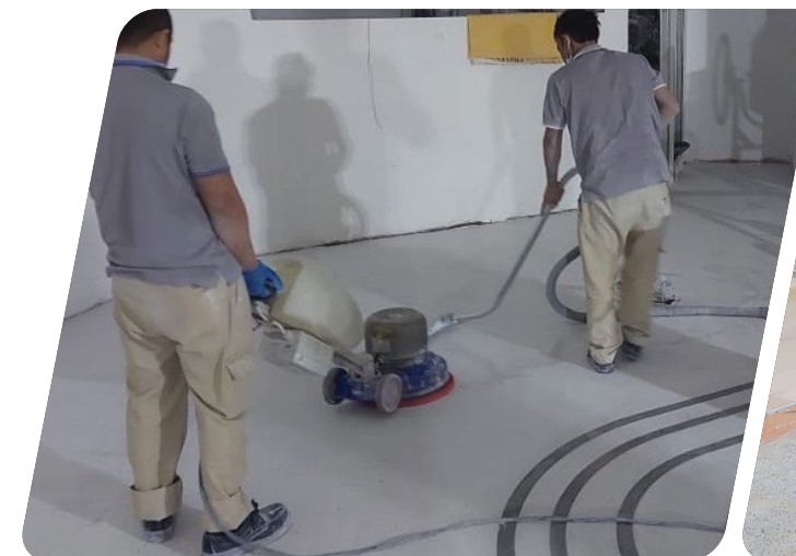
7 Polishing & Buffing Polish and buff the surface using a light weight polishing machine
