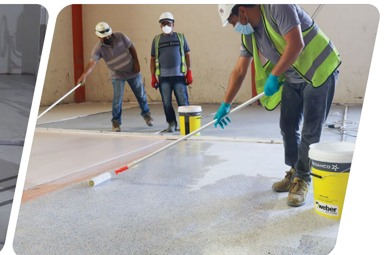
8 Sealing Seal the surface with weber euroflor Seal S
