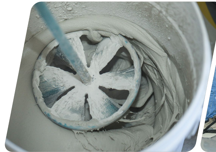
3 Mixing Add weber euroflor Design to the pigmented water and mix for 5 minutes
