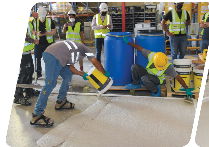
3 Pouring Pour the mixed components wet on wet into the floor
