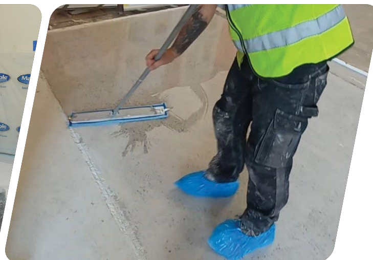
6 Filling & Hardening Apply weber euroflor Fill to fill the pin holes then followed by weber euroflor Protect to harden the surface
