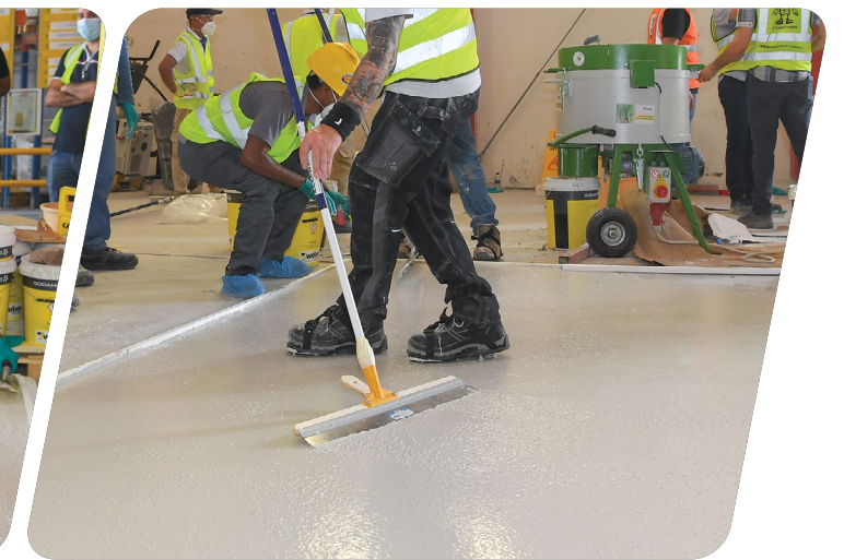
4 Levelling Level the mixture by using a smoothing leveller tool
