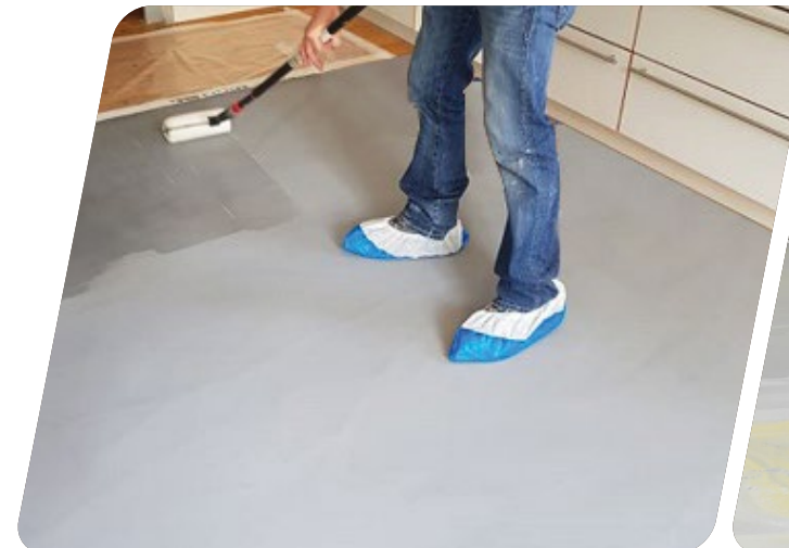
7 Sealer Seal the floor with weber euroflor Seal
