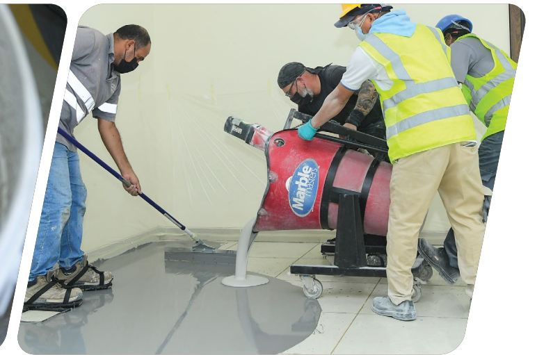
4 Application Pour the mixed product into the floor
