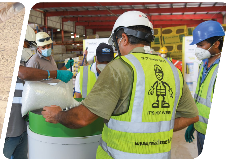
2 Pigmentation Mix weber euroflor Terrazzo binder/ filler and terrazzo aggregates with clean and cool water
